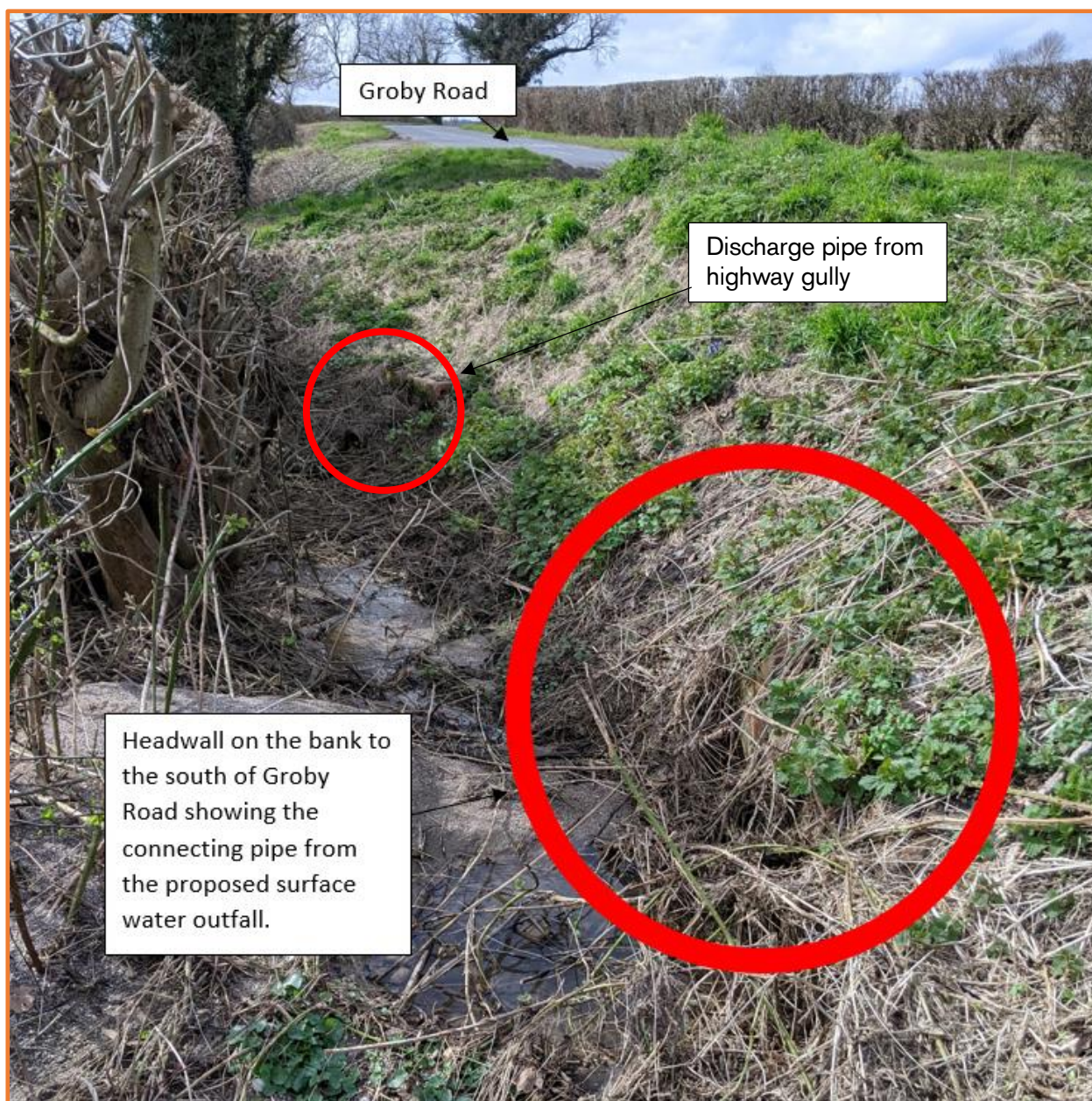
Figure 1: An image demonstrating the connection between the proposed surface water outfall and the drainage network to the south of Groby Road.
