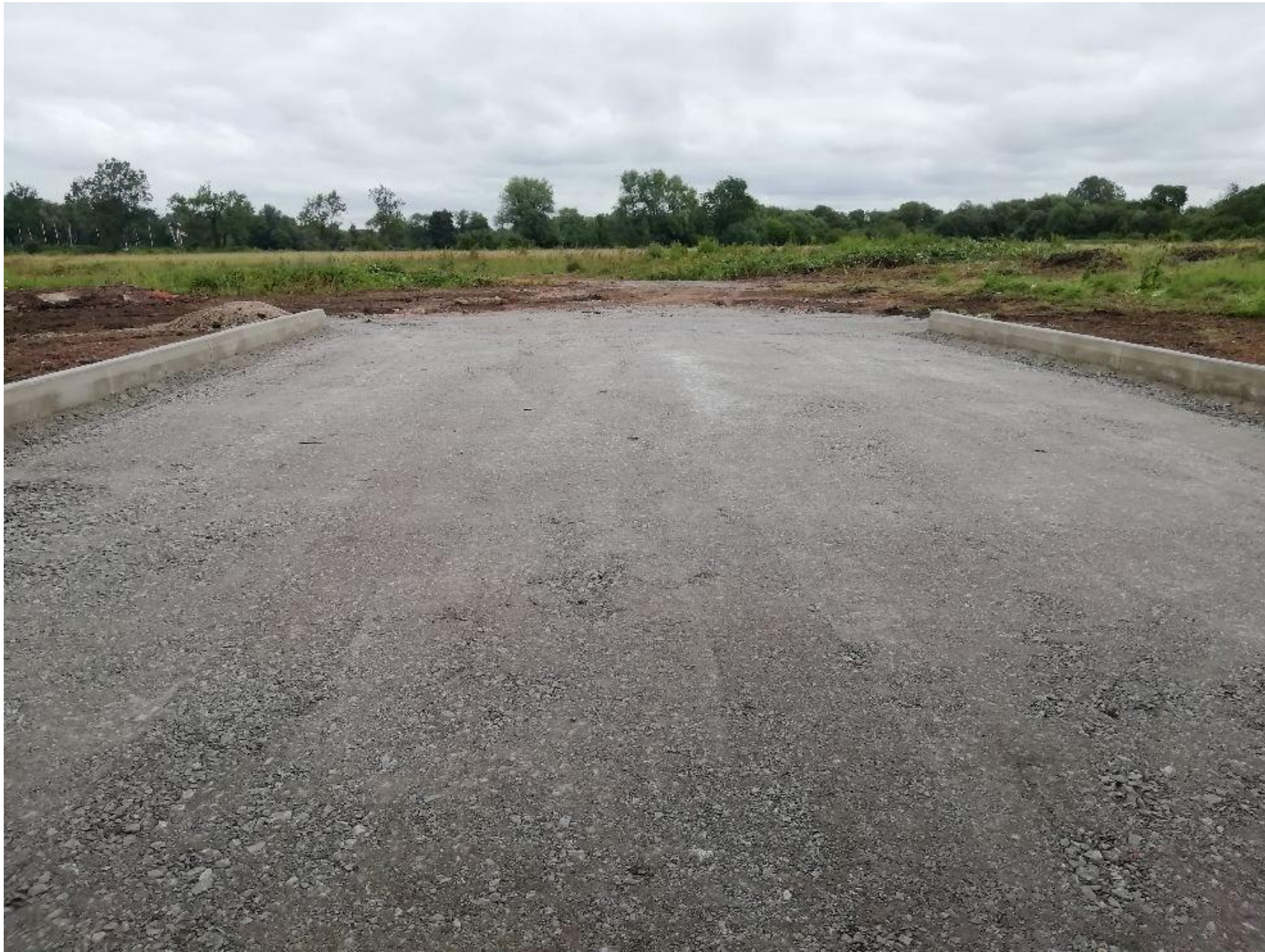
Figure 1 – Hardstanding laid at the main site entrance, from High Street.
