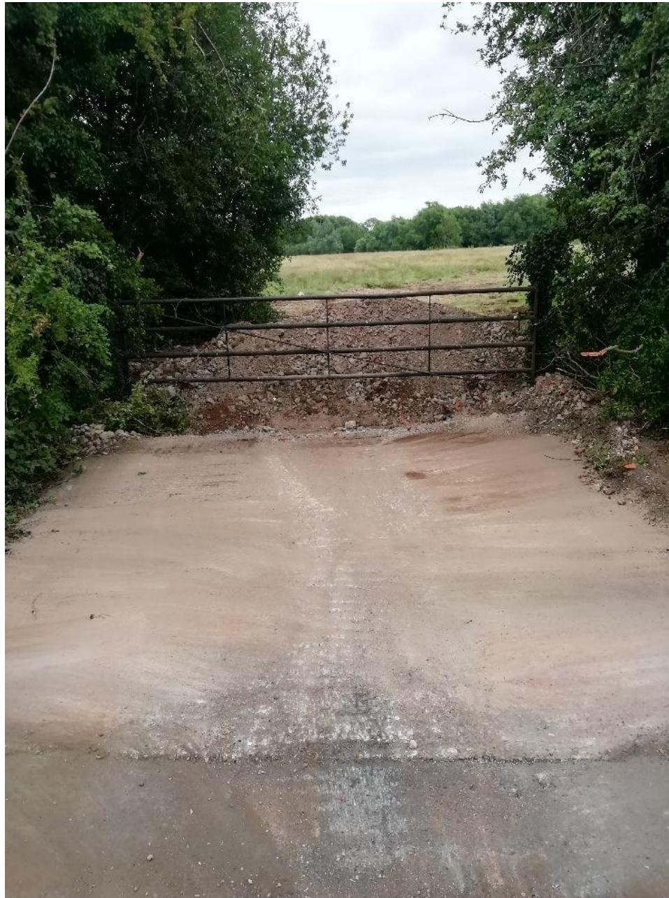
Figure 4 – Hardstanding laid at the site entrance from Fosse Way.
